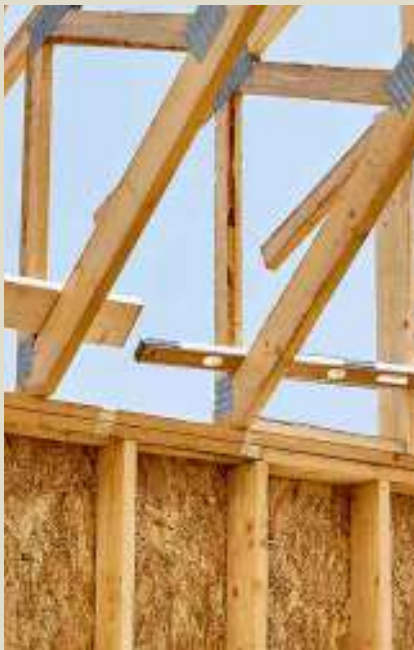
Build Engineering Spaces for Tomorrow
